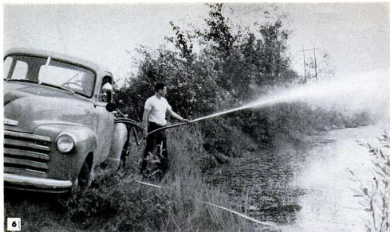
Here water is being pumped from the farm pond. Note the long suction line. Throws stream more than 60 ft.
